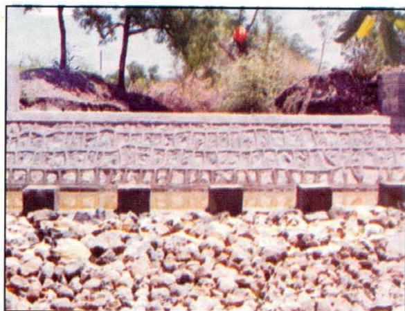
Plate 8. A view of stop dam constructed in watershed area.
